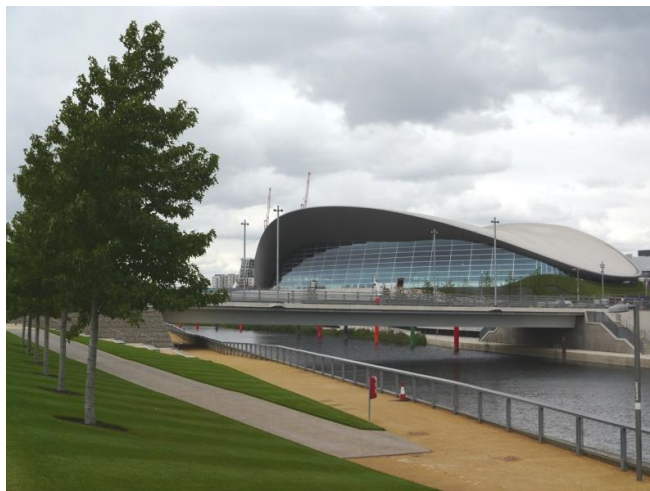
Work underway on the Legacy Masterplan in The South Park. Queen Elizabeth Olympic Park
