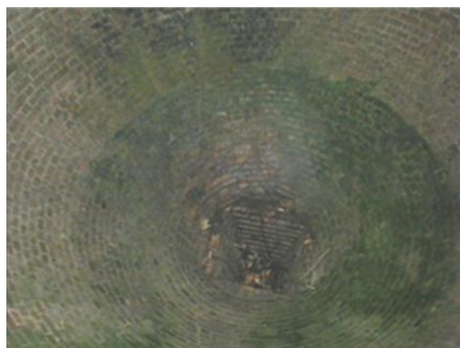
Below: Conical shape brick chamber, icehouse Rode Hall
