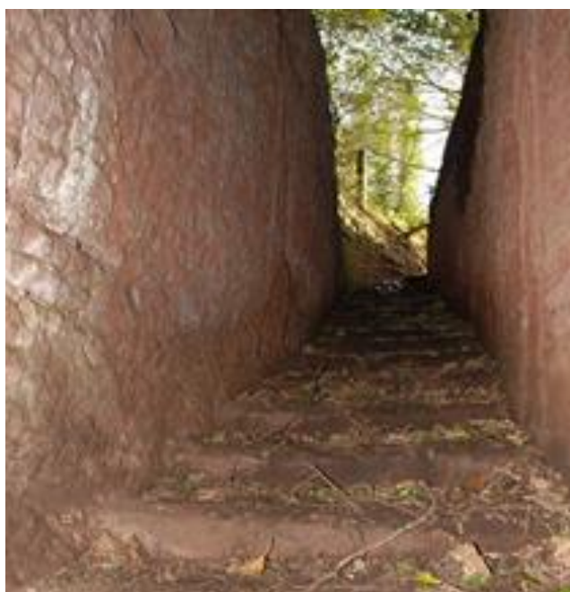
Burton Manor, steps to N entrance of icehouse
